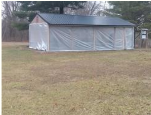
Shelter house wrapped and ready for DELARA's WFD activities.
